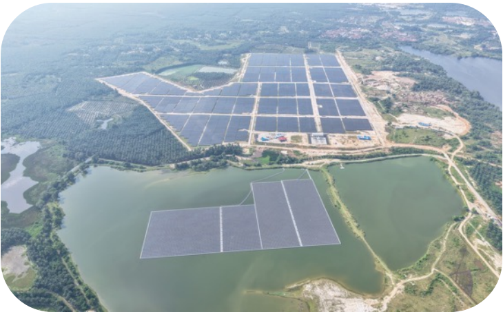
CGPP Solar Farm
