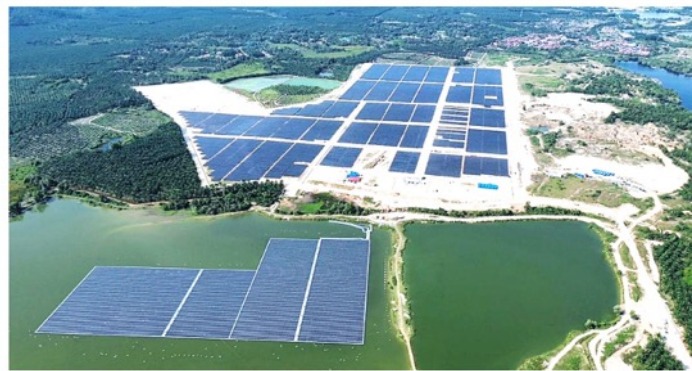
CGPP Solar Farm
