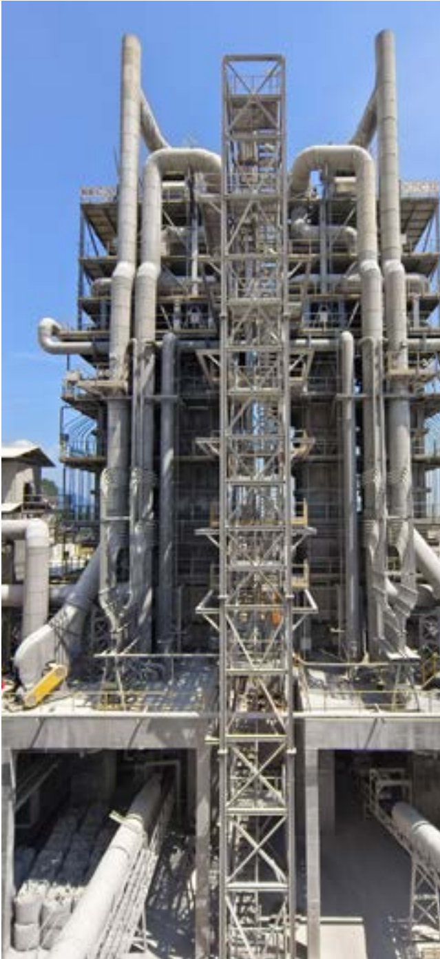
Lime Kiln Location: Gopeng, Perak
