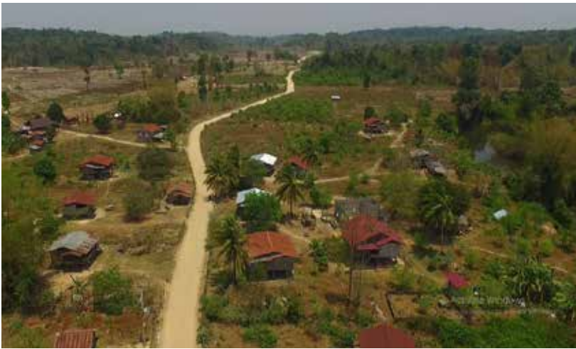
Road expansion project at Nong Ping village, Pathoumphone district, Champasak province.
