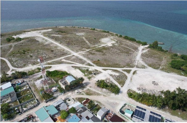
An aerial shot of our solar site in Hinnavaru, Maldives.
