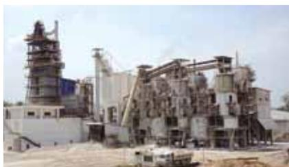
A new lime kiln and downstream processing plants were commissioned in August 2015 while another new lime kiln will be commissioned in the fourth quarter of 2016, boosting capacity significantly. Development works are being undertaken in preparation for the addition of another five kilns in the near future.
